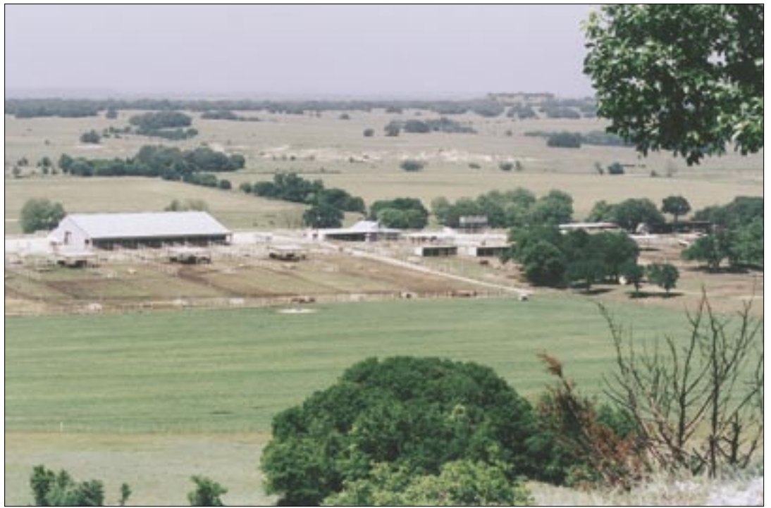
W4 Ranch encompasses 12,000 acres of native grasslands, water sources and improvements. The Walker family spent years developing the infrastructure and buildings in order to have a functional, working cow ranch.
